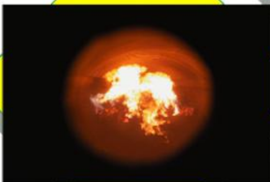
Inside the Combustion Zone
