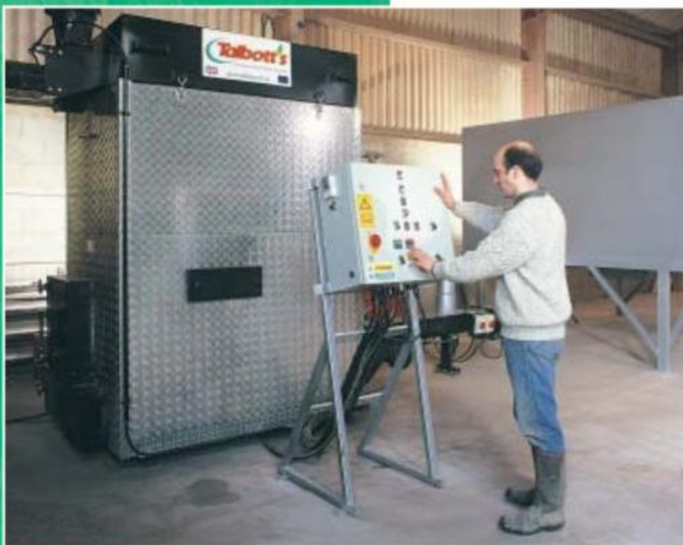
Above: Gareth putting his investment to use, using the biomass combuster to heat the Paddock House Farm complex.
